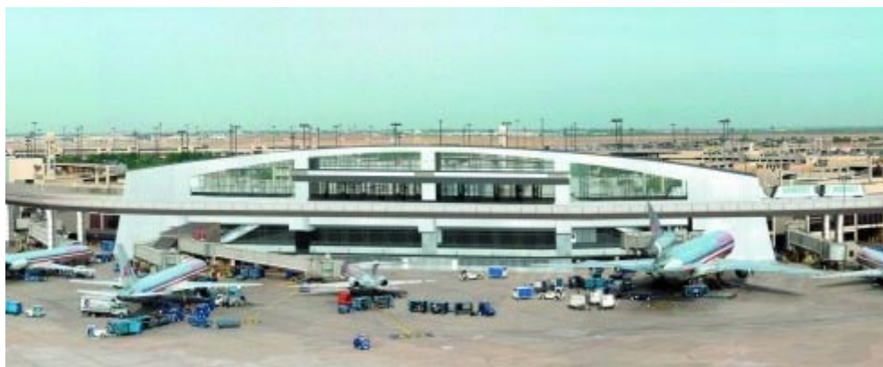
The APM system includes 12 center-platform stations, two at each terminal. The columns are spaced at 90 ft (27 m) on center to conserve valuable airfield space. The twin guideway lanes split and run along the sides of each station, supported by the station framing.
